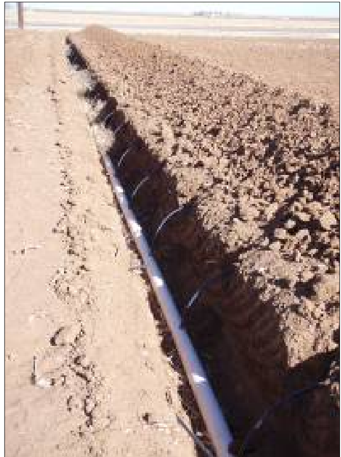
Figure 6: Drip tape laterals were shanked into the ground and connected to PVC submains at Jordan Farms.
