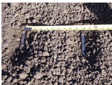
Tape is placed 10 inches apart, about 0.5 – 1.0 inches deep.
