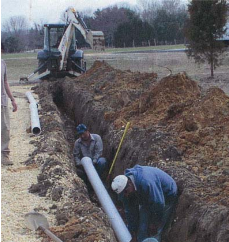
Workers install irrigation pipeline, financed via the EQUIP program.
